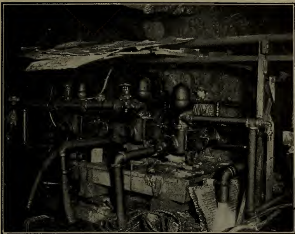
Battery of Cameron Pumps installed in "Belmont" Tunnel, under East River, under Man-O'-War's Reef.
